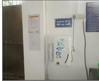
External photo(s) of the production unit(s) Drinking Water Point .JPG
