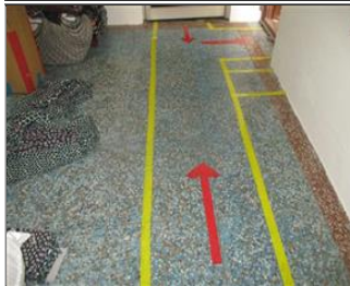
Photo of fire safety equipment Aisle Mark with Direction Sign.JPG
