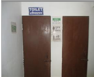
Photo of the inside of the main production hall Toilet View.JPG
