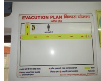
Photo of non-conformity Incorrect Evacuation Map for Direction.JPG
